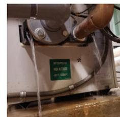
CEM dismantled the heater to inspect the heater inlet and outlet tubes.
