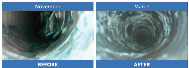
*“Worth noting are the piles of debris seen in some of the pictures. This is scale flake that had fallen off of the tube and was in the process of rolling out of the heater until it became lodged.”*
